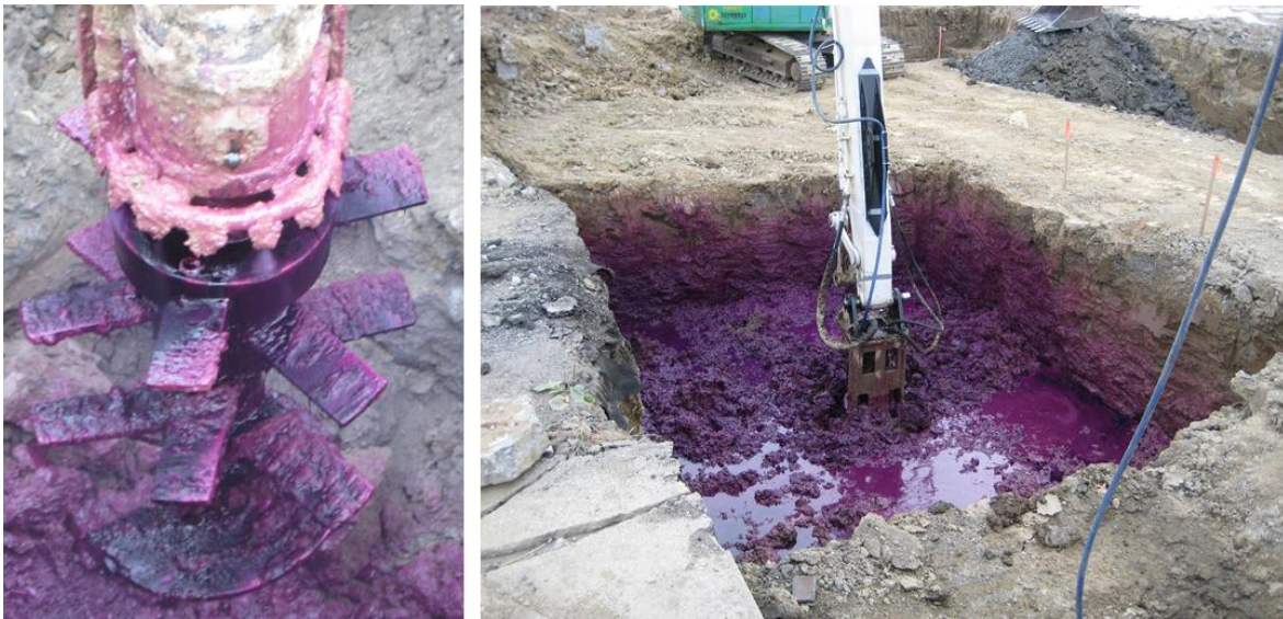
Figure 1. Example of soil mixer used for environmental remediation
