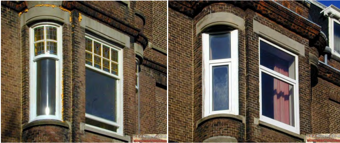
Figure 1: Replacement of single glazing in a wooden window frame by standard double glazing in a plastic window frame. Photographs: E.J. Nusselder
