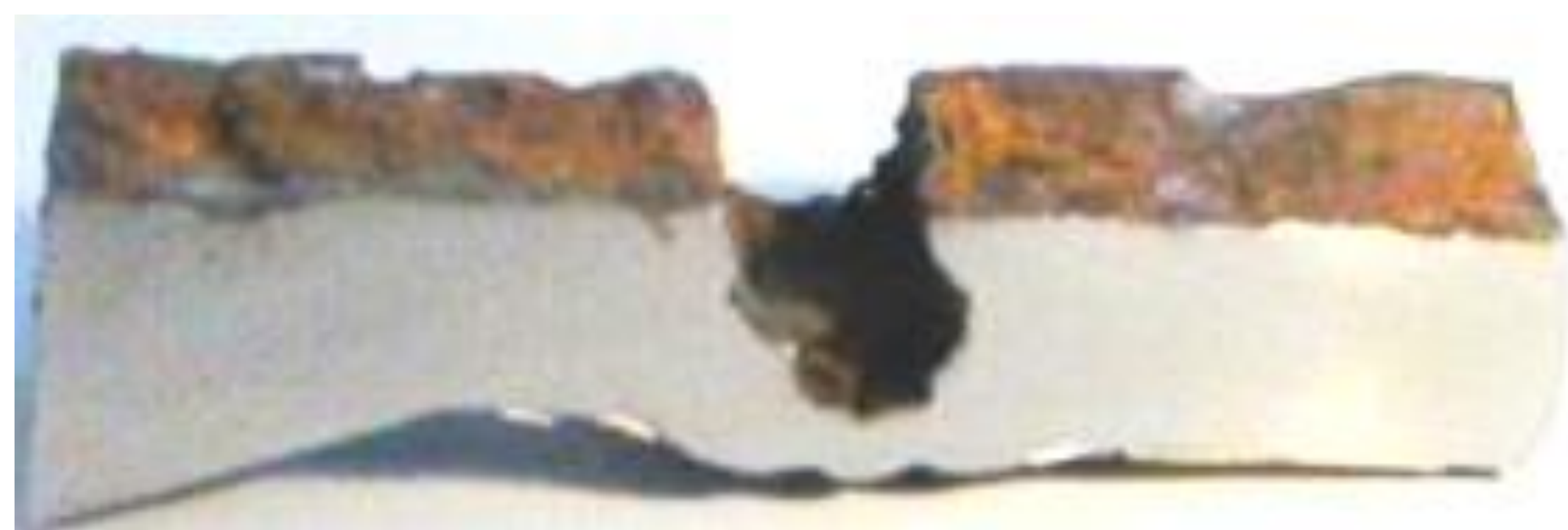
Fig. 1. Corrosion of the welded joint
