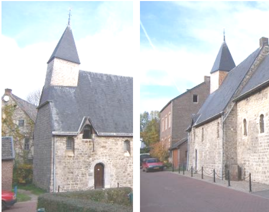
Figure 1. The exterior of the church of Lemiers (Source: nl.wikipedia.org 2012).
