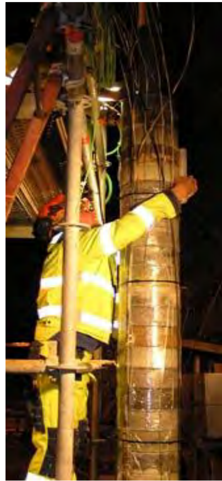
Installation of the package
